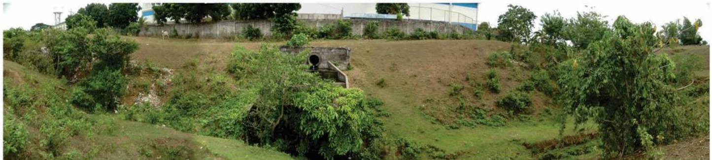
3 - Drainage outfall inside the property
